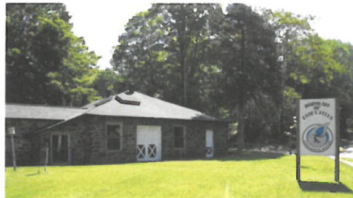
Pumping station on Runnymede Road
