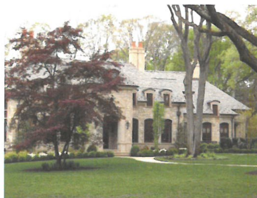
Replacement of historic structure on Oldchester Road
