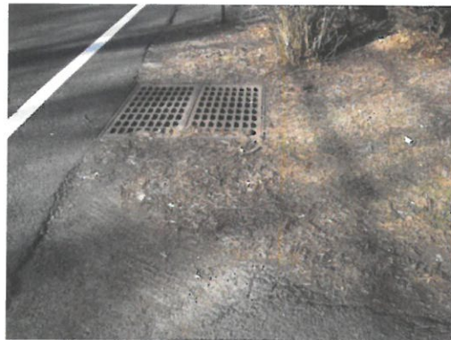
Storm sewer on side of roadway
