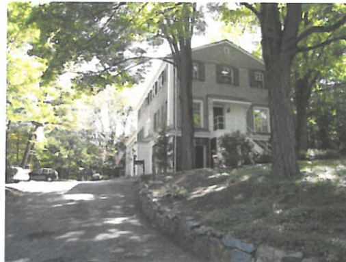
Non-conforming commercial use off Runnymede Road
