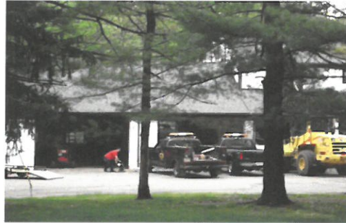
Service Building and the Public Works Department
