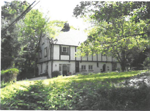
Multifamily dwelling on Oak Lane
