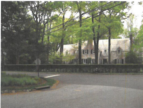
Residential dwelling on Oval Road
