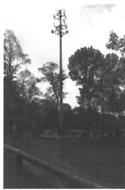
Cell tower in Roseland
