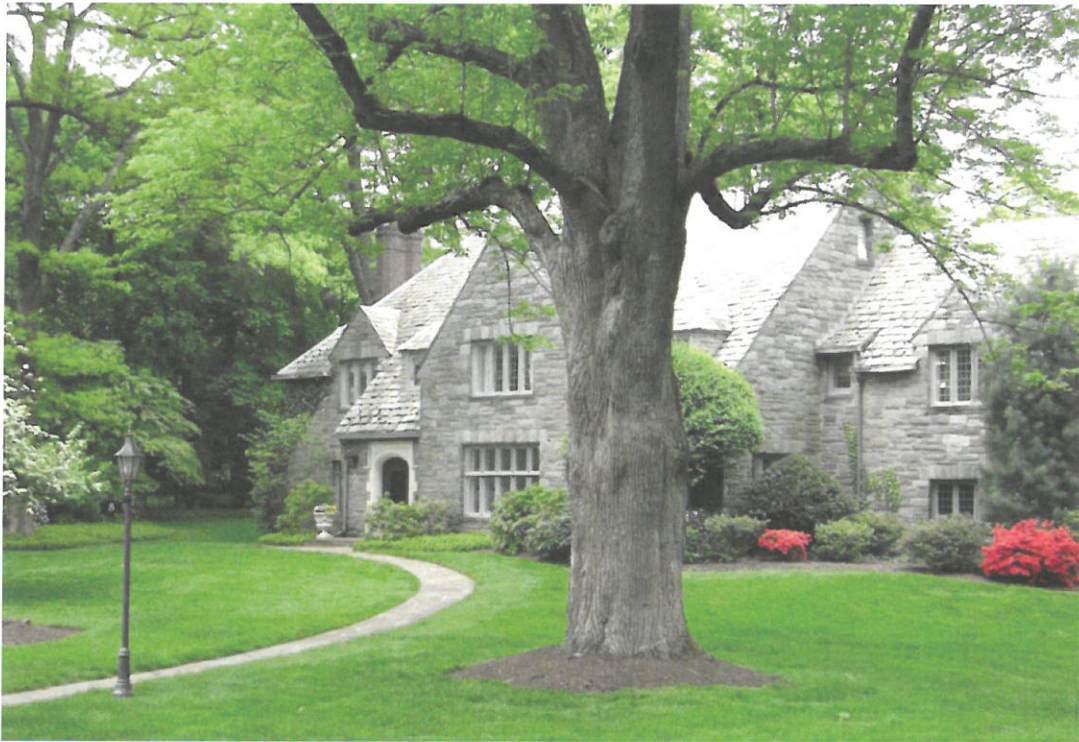
Residential dwelling on Beechtree Lane
